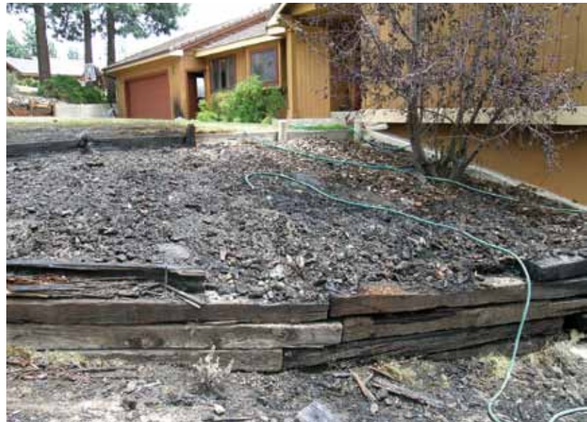
▲ Figure 1. Embers from an oncoming wildfire ignited the pine bark nugget mulch in this flowerbed. The burning mulch then ignited landscape timbers and scorched the adjacent lawn. Fortunately, the house was separated from the mulch by lawn and a concrete sidewalk.
